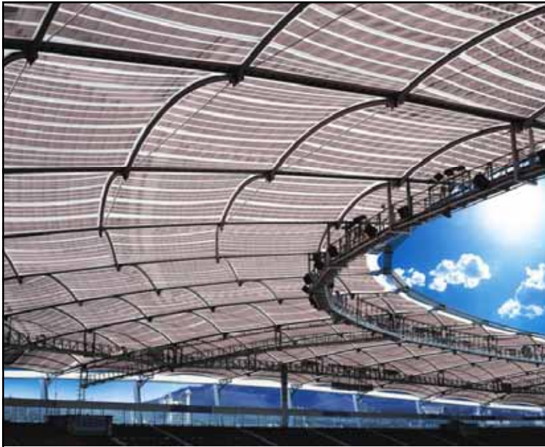
Gottlieb-Daimler-Stadium, Stuttgart, Germany (including PV, Computer Rendering) © SolarNext AG/ Hightex Group - IFAI Presentation - Dr.-Ing. Jan Cremers - 13.06.2008
