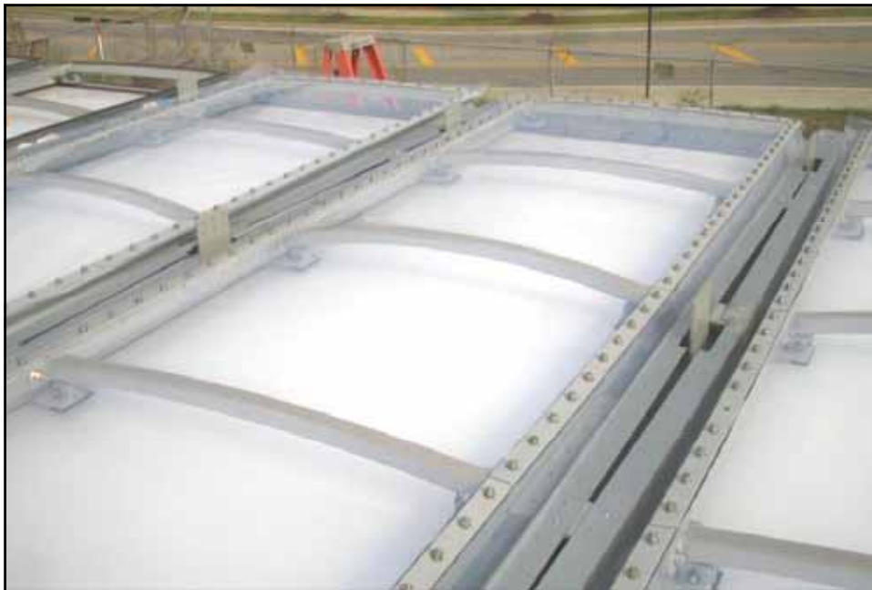
Project in the US with translucent Aerogel-filled ETFE-Roof-Panels, U-Value < 0,25 W/m 2 K © SolarNext AG/ Hightex Group - IFAI Presentation - Dr.-Ing. Jan Cremers - 13.06.2008
